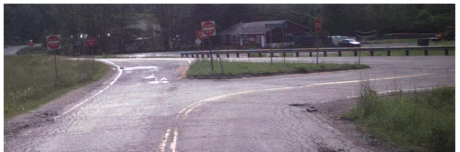
Example of centerline markings that follow the curvature of the road
