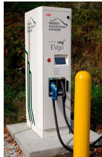
A DC Fast Charger with two charging plug types, one on each cable.
